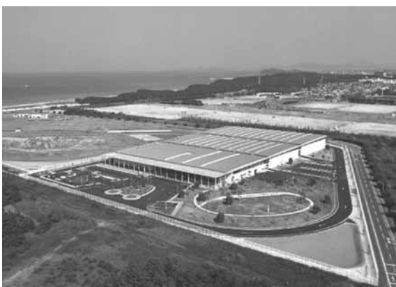
Fig. 1 Fukuoka Uminonakamichi Nata Sea water Desalination Plant
