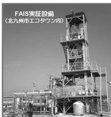
Fig. 1 Image of the 2 t/day-capacity demonstration plant
