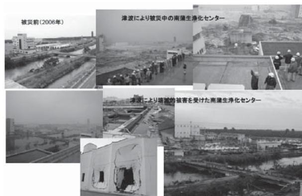
Photo. 1 The Damages of Minami-gamou sewage plant in Sendai city (Japan MLIT)<sup>2)</sup>
