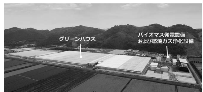
Fig. 1 Overview of SARA's greenhouse and biomass power plant
