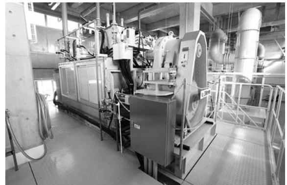
Fig. 6 The Shaft Sliding Screw Press Dehydrator
