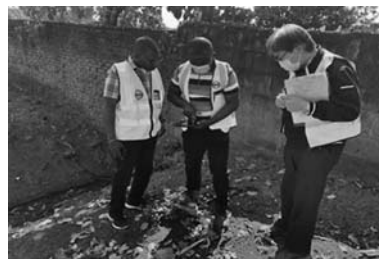
Photo. 1 On-site work to check water meters
