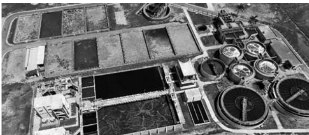
Fig. 2 Full view of Salori sewage treatment plant, Allahabad, Uttar Pradesh, India
